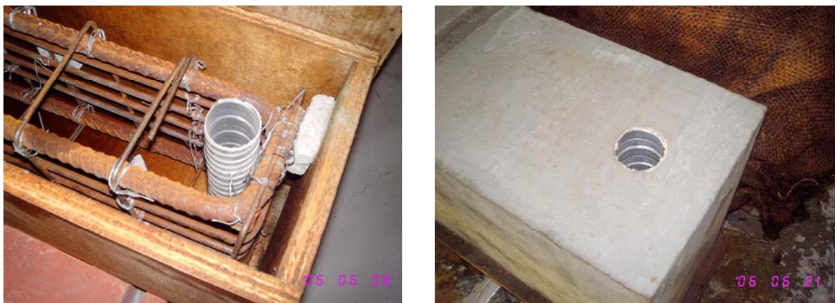
Figure 11 Preparation of sleeve in precast beam
