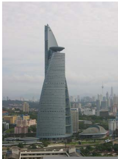
Fig. 2. Telekom Tower, Kuala Lumpur, Malaysia.
