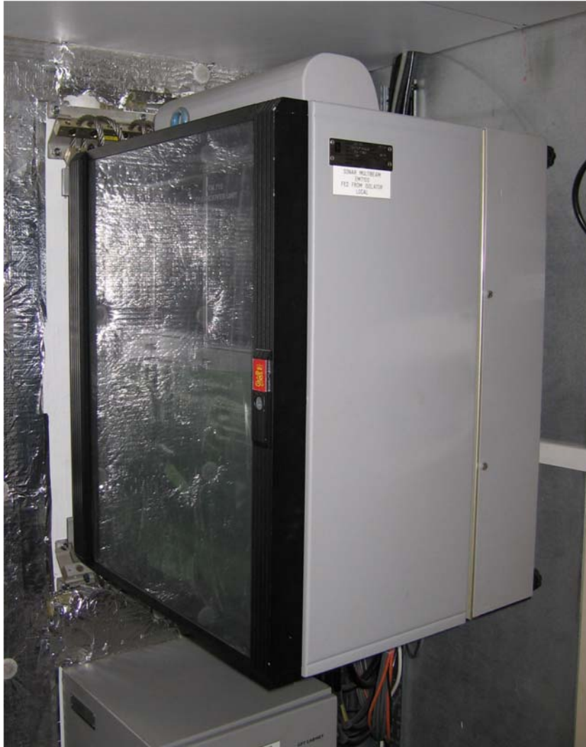
Figure 13 Installation of the Transceiver Unit on “HMS Endurance”
