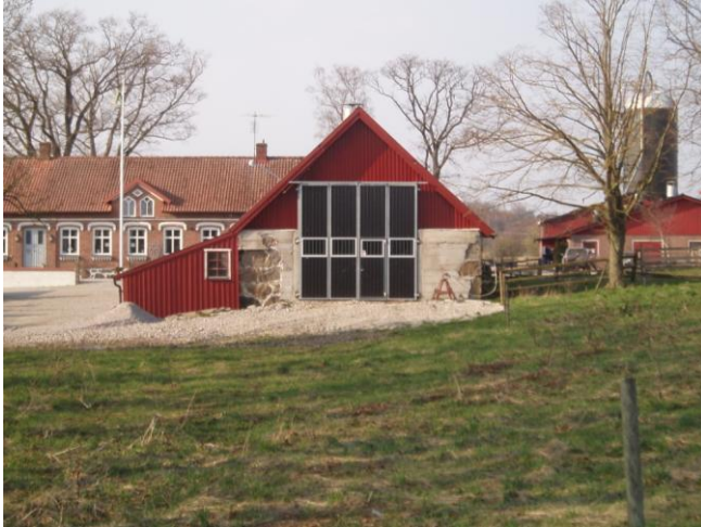
Figure 15. Example of a traditional agricultural building converted for the use of modern, large machinery. Functional thinking before aesthetics, the destruction of the traditional AB's proportions and its original cut-block stone material replaced with reinforced concrete and an aluminium-reinforced plastic folding-door.
