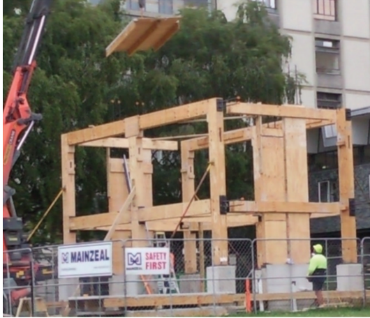
FIGURE 3: Reassembly of experimental building with TCC floors within the University of Canterbury campus, now known as the EXPAN building.
