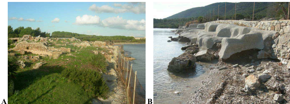
Fig. 3.6 - A) Fence installed around the site. B) Stabilization of the structures directly in contact with the sea.
