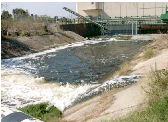
Figure 4.37. Canale delle acque basse and pumping station.
