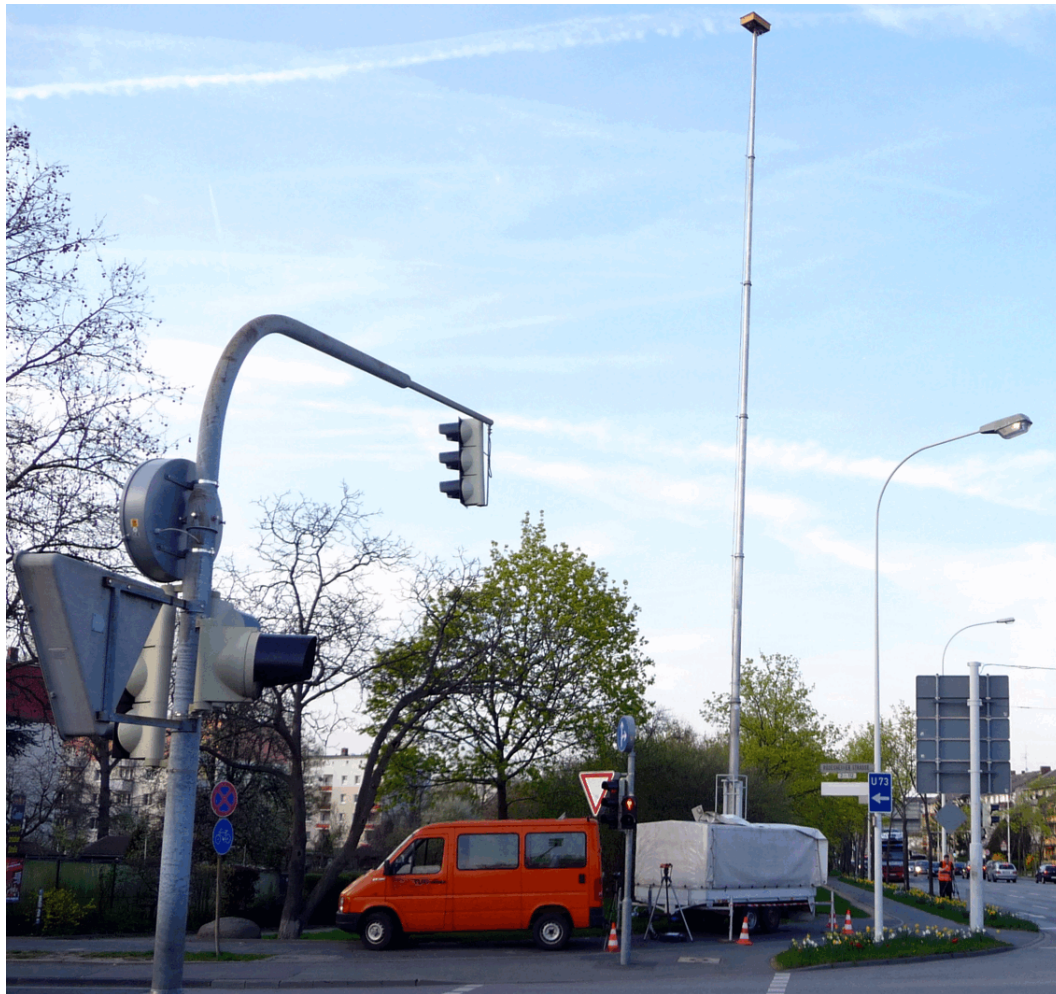
Figure 19: Extension mast located next to an intersection
