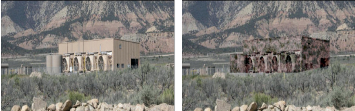
Figure 36: Two stages of a camouflaged Building.
