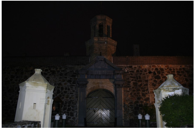
Ill. 6: Castle Gate of Cape Town Castle (photo C. Comoli 2008)
