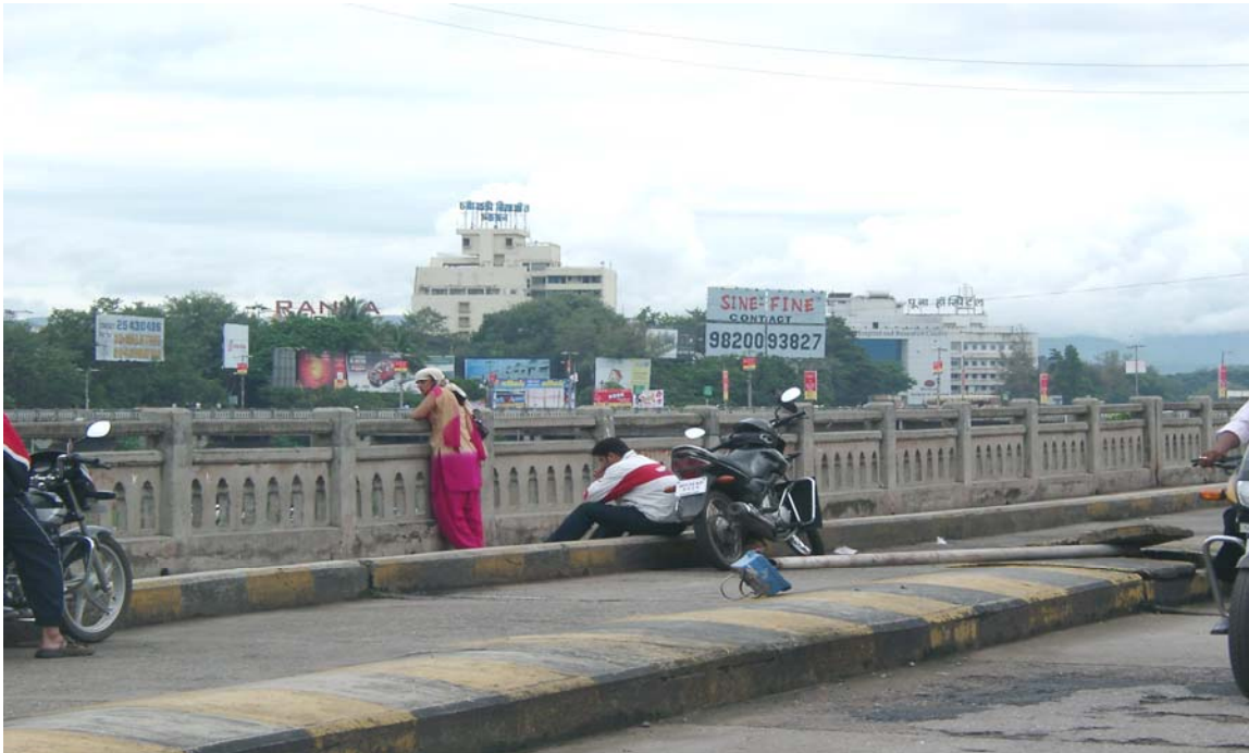
Figure 12: Photograph of Z-bridge 1 441
