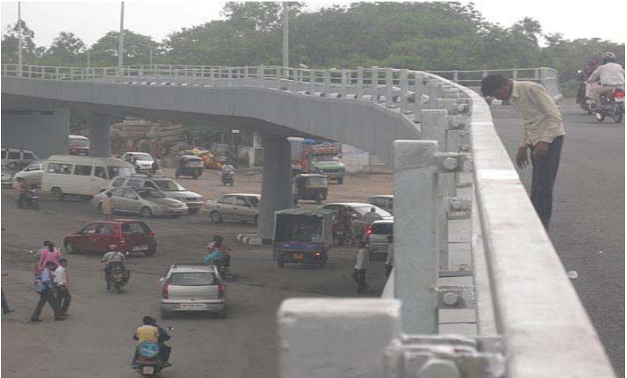
Figure 7: Photograph of the fly-over bridge at the Pune University chowk 313
