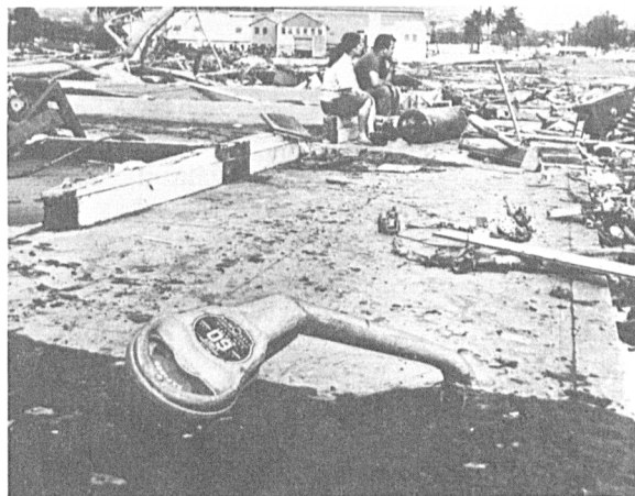
FIGURE 1. Destruction wrought by the Chilean tsunami of 1960 at Hilo, HI
