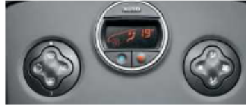
control of air-conditioning (left), air-conditioning display (center), control of ventilation (right)
