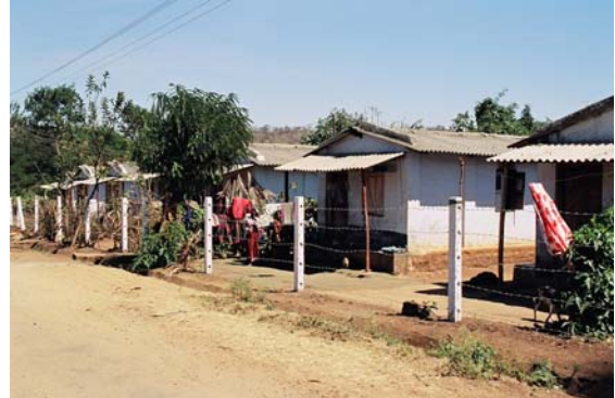
Figure 19 Adivasi houses constructed by the government, Eruru village The corrugated iron roofing of these houses is completely unsuitable for (semi)tropical climates (9. focus group interview 2007). Photo: C.C. Aufschnaiter
