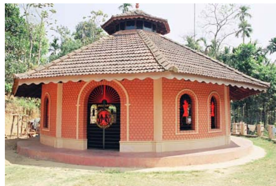
Figure 34 An Adivasi assembly house TUDI (Tribal Unity for Development Initiative), Panamaram, Wayanad District, Kerala (2. semi- structured interview 2007) Photo: C.C. Aufschnaiter
