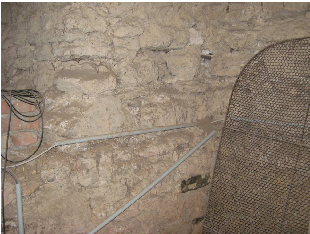
Abb. 154: Hollenburg - Turm, 1.OG, Westwand, Baufuge
