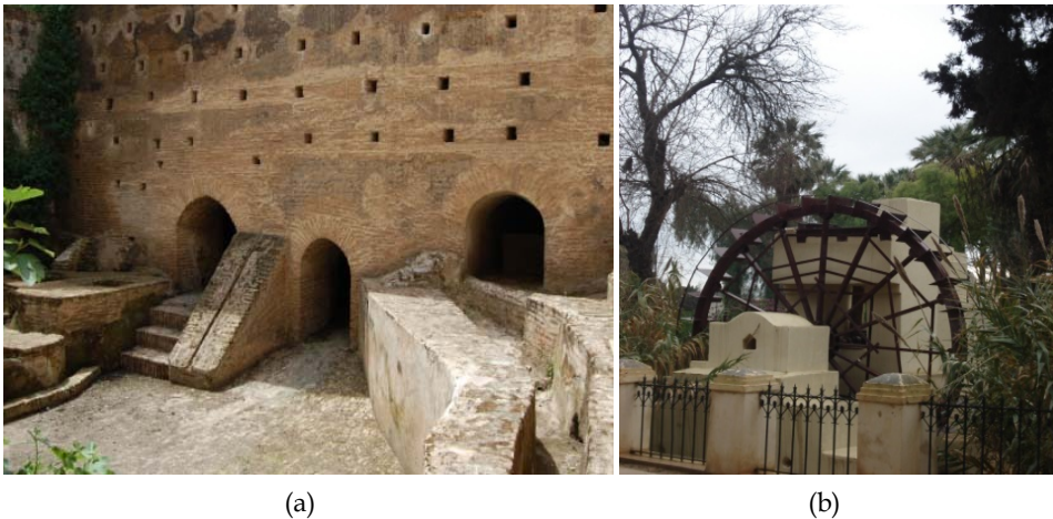
Fig. 5. a) Water distributor, Fes b) Noria from which the water flowed to the distributor
