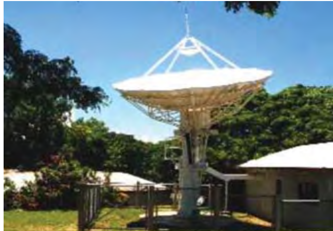
Figure 2. Antenna at Hub Station in the Fiji Islands
