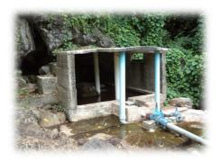
The WAF supplies water from the Mua catchment which is located approximately 20 kilometers from Naselesele village (Figure1). The water source is spring water which is directed into a holding cement pound of 5m (L) x 3.5m (W) x 0.5m (D) in size. This water is pumped 8.4 kilometers into a 50,000 gallon cement water tank for treatment through chlorination drip method. This treated water is pumped 5 kilometers into two 26,000 gallon cement water tanks at Naselesele
