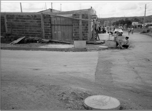
Figure 1. Simplified sewerage installed in a low-income urban area of the Federal District, Brazil
