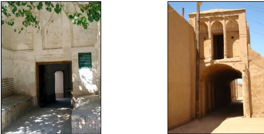
Figure 2: The 'SABAT' (simple and beautiful half covered passageway) as a public space. Boshrooyeh city (Author)
