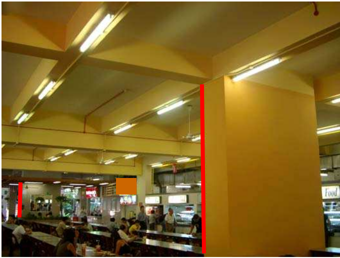
Figure 8a - Singapore Polytechnic floor viewed from below, with near and far columns highlighted
