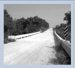
Look at loads. Accumulated gravel surfacing and bituminous overlays sometimes get carried over the bridge deck to improve the ride. If their weight has reduced the bridge's capacity for carrying traffic loads, consider removing the extra surface material to improve the bridge's durability and load-carrying ability.
