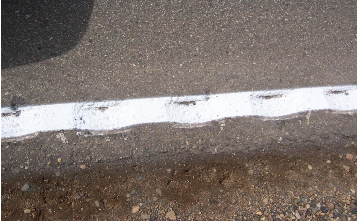
Figure 1.1. Completed edge-line rumble stripe on a rural highway in Iowa
