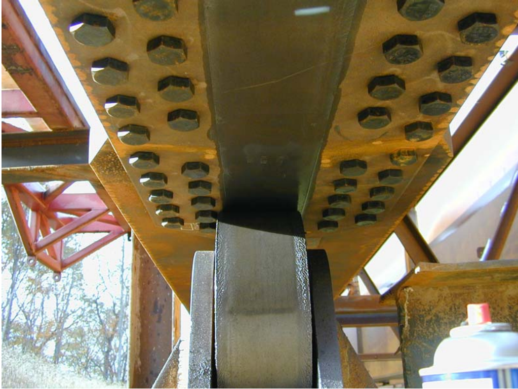
Figure 3.7. Vertical roller positioned between bottom flange splice plate bolts
