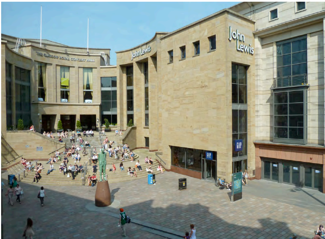
Fig. 1: The entrance to the Royal Concert Hall with the semi-circular square. The windowless stone-clad front and the large windows on the right belong to the shopping centre Buchanan Galleries (author's photograph).
