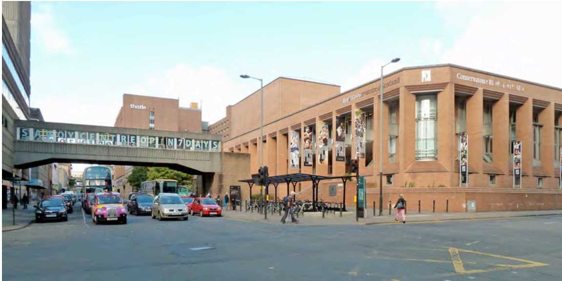
Fig. 16: The Royal Scottish Academy of Music and Drama (1983-88, now renamed Royal Conservatoire of Scotland), designed by Leslie Martin. The surroundings betray some of the debates over urban form. The grey cast-concrete overpass leading to the shopping centre Savoy Centre (opened in 1973) is a relic of the 1960s plans of a layered city where streets are reserved for cars and pedestrians move on elevated decks. The cube on the overpass's right end contains the stairs leading down to the pavement. Only this part of the bridge was clad with the same clinker brick as the Royal Academy building, making the clash between the two urban concepts visually apparent. Together with the canopied bicycle stands (built in the 2000s) it represents the post-1960s model of the mixed-traffic city.
