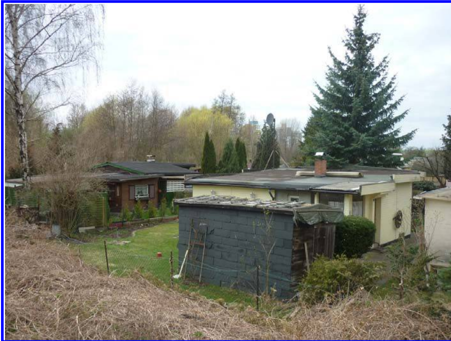
Figure 23 Improved construction, Am Segelluchbecken allotment colony next to the Märkisches Viertel (author's photo, 2011)
