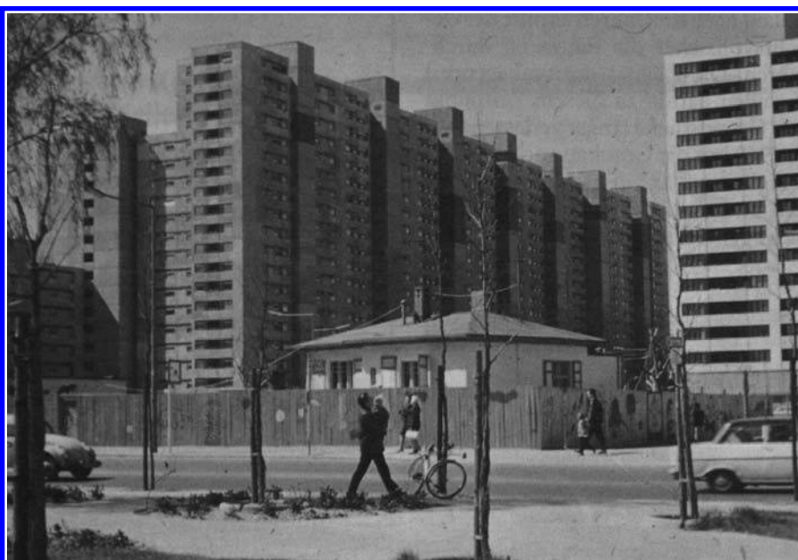
Figure 22 Haus Genzmann on Wilhelmsruher Damm and Treuenbrietzener Straße in the Märkisches Viertel, 1971. The building was later demolished (Hildebrandt and Schlickeiser, Abschied von der Laube , image no. 365)
