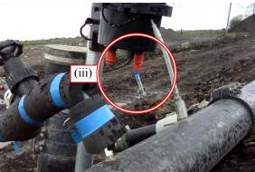
Figure 4: Site-specific issue rectification (i) Waterblockage, (ii) Tube shrinkage, (iii) Connection breakage due to pipe collapse
