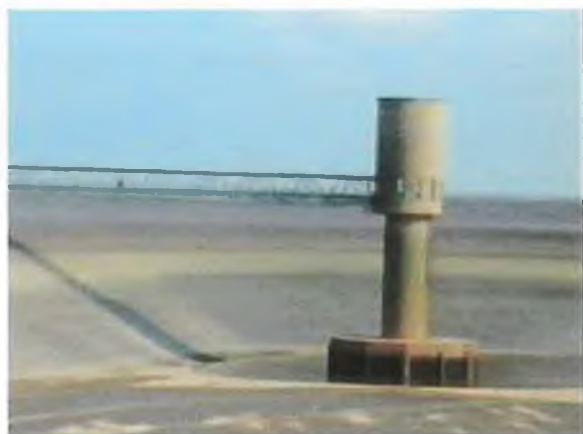
Figure 84: Ardnacrusha Power Station, in C Oblique O (© Blue Funk, 1999)
