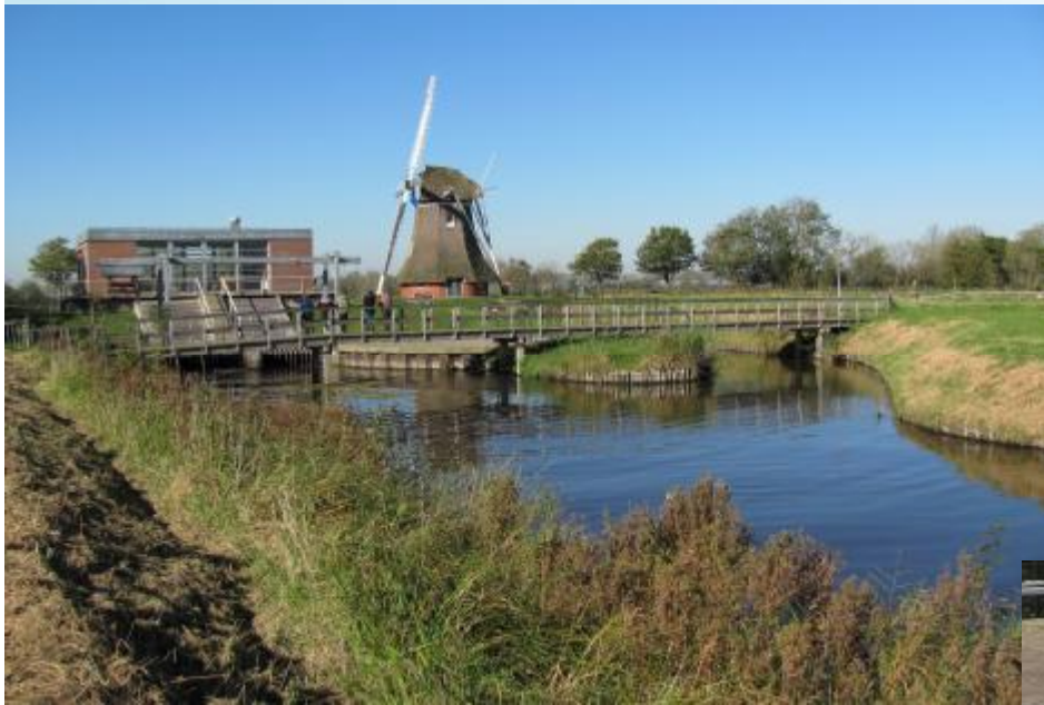
Caspar Hommes Pumping Station near Groningen, Netherlands
