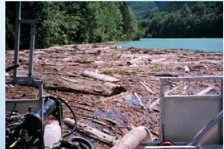
Debris crowds the work barge downstream. Note the motive water hoses and motor. Once the FVES is activated, debris mass begins to move and remains in constant motion while FVES runs. BPA Test on Cowlitz River, 2008
