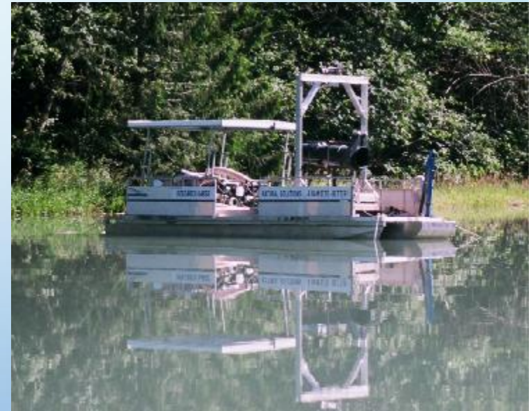
NS work barge on Cowlitz River
