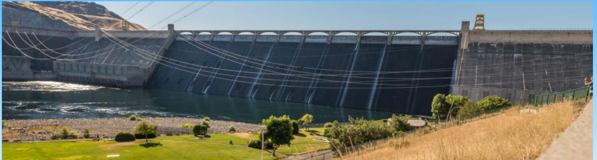
Grand Coulee Dam, Columbia River, Washington
