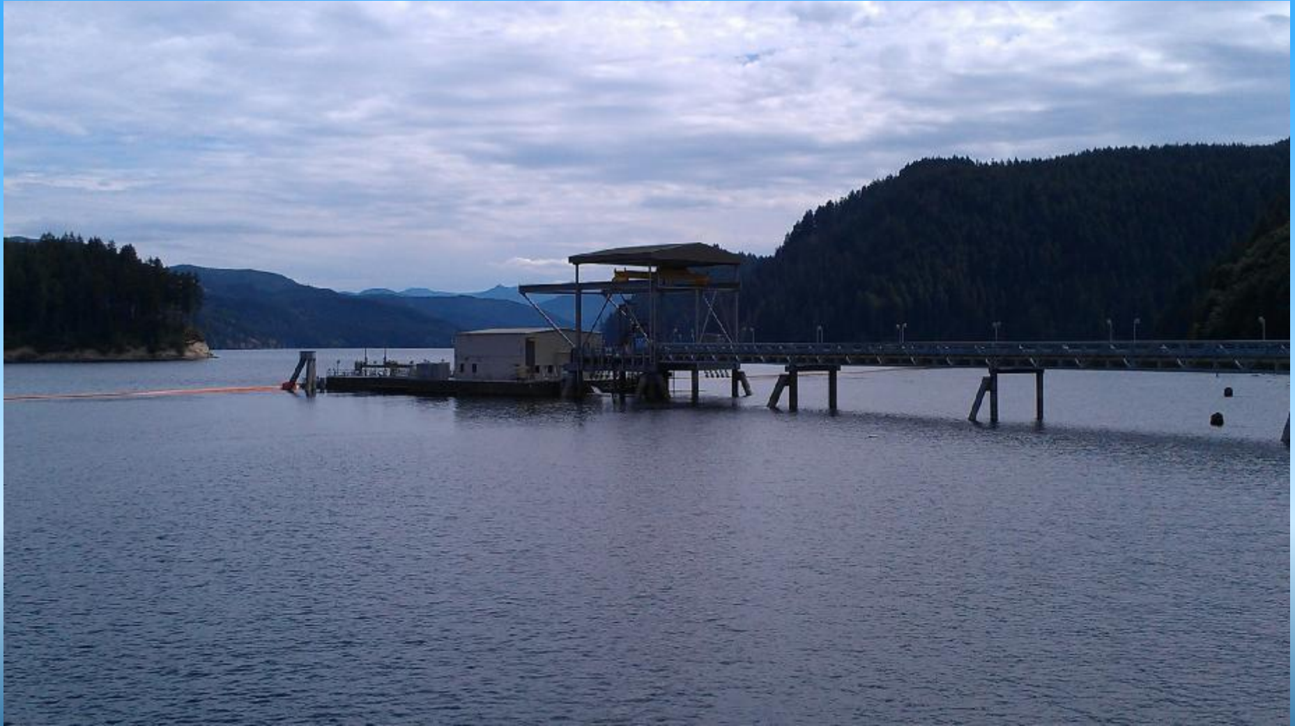
Swift Dam Fish Collector, Lewis River, Washington
