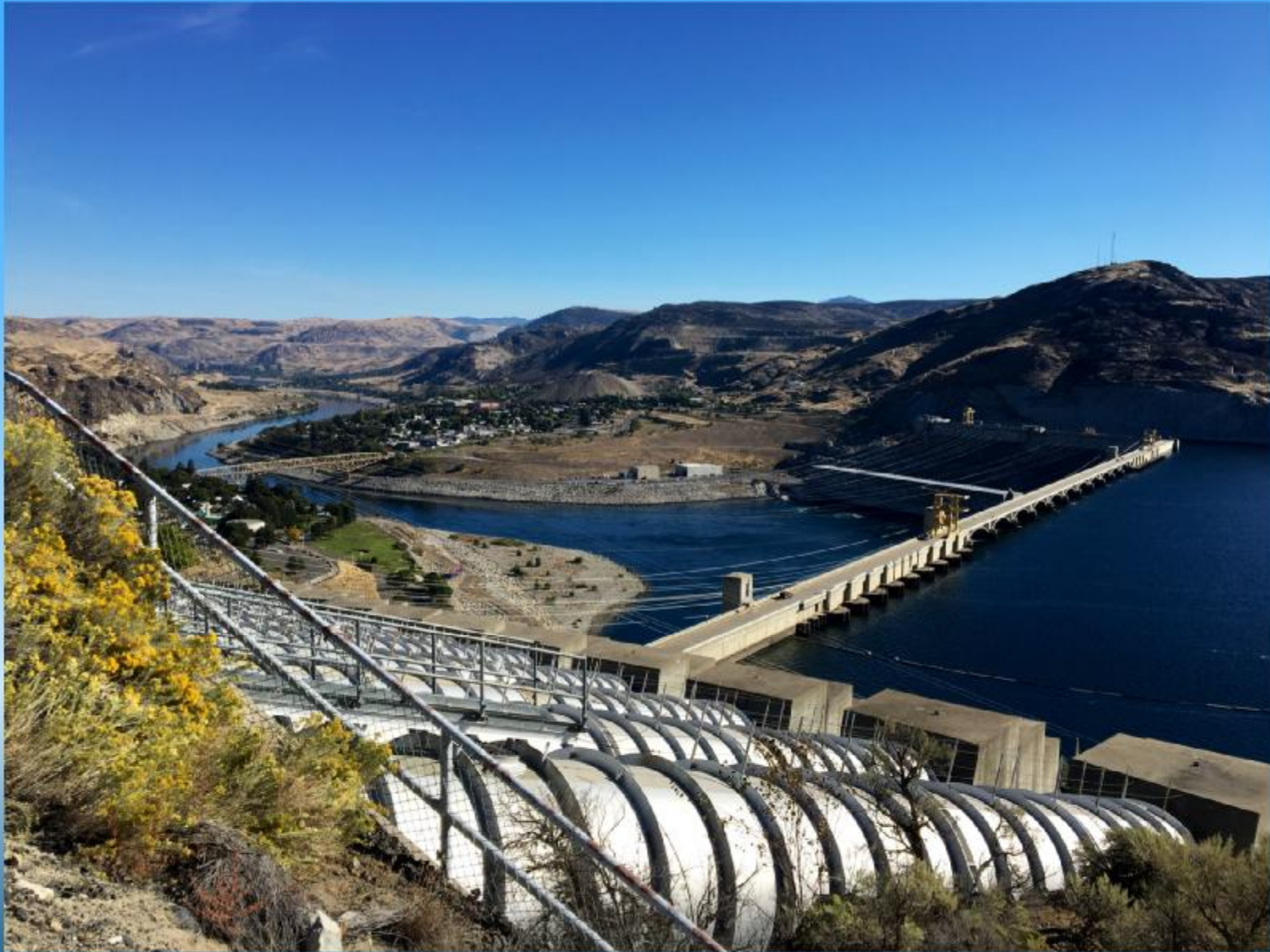
Grand Coulee Dam, Columbia River, Washington
