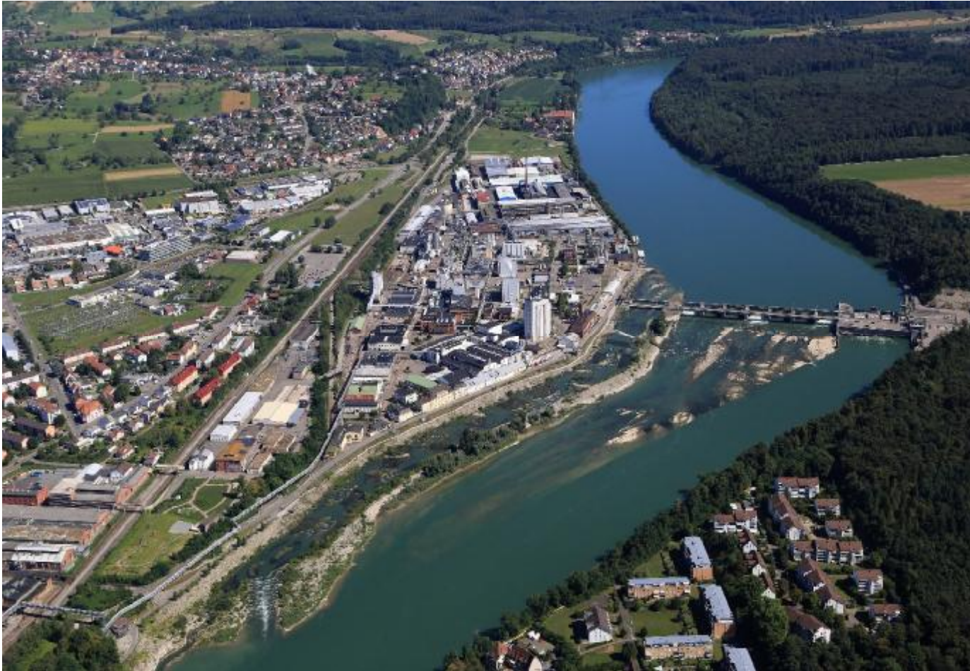
Hydropower plant Rheinfelden (discharge capacity: 1500\text{m}^3/\text{s} , installed capacity 100 MW)
