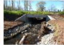
SR 99 at West Fork Hyalison Creek after the old culvert was replaced in 2015, restoring access to over 2 miles of upstream habitat for dunn and coho salmon, steelhead, sea-run cutthroat, and resident trout.
