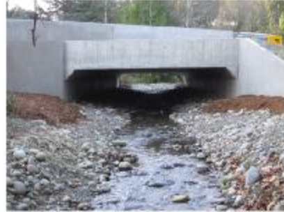
Stream Simulation Culvert
