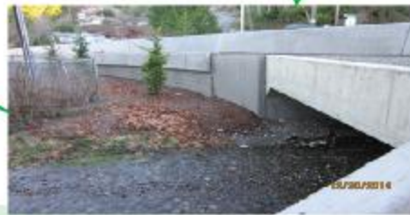
After – new 20 foot (6.1 meter) box culvert
