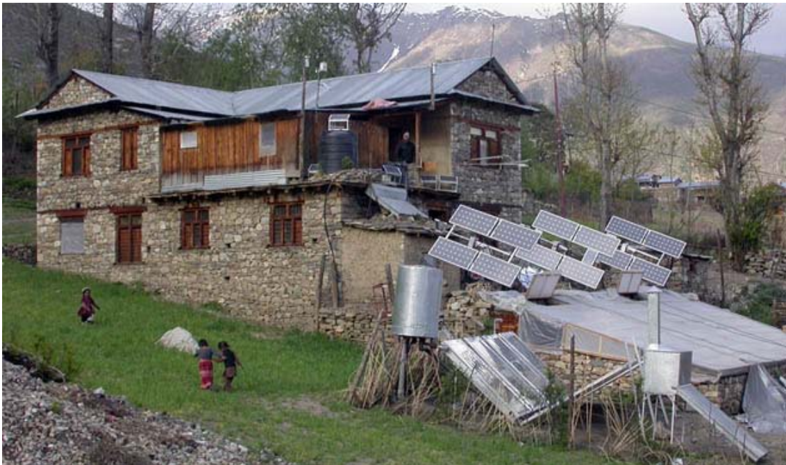
Fig. 2: RIDS-Nepal Simikot office in Humla Nepal at 3000 meter altitude, with a 900W P monitored Solar PV system. The system is monitored in detail since 2004 for its performance throughout the years.
