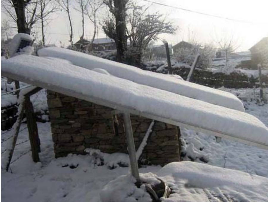
Figure 14: In Humla, it is not infrequent that during the 4 winter months from November to February snow covers the solar PV array fully.
