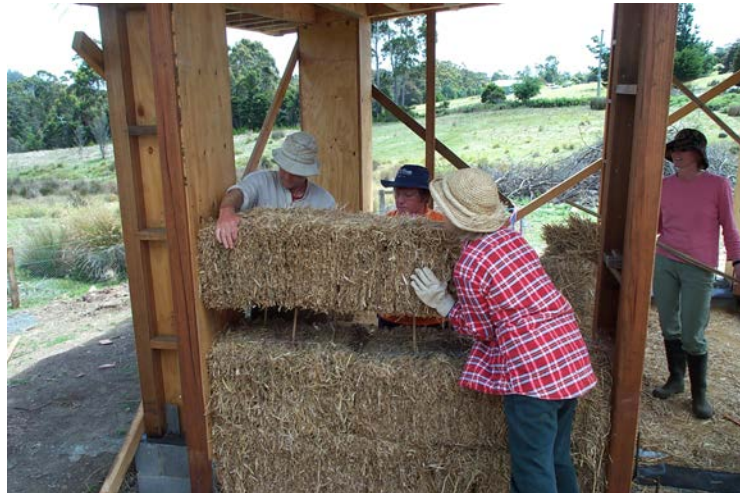
Image 11-10 Community building workshop: staking bales (Parnell, 2002)
