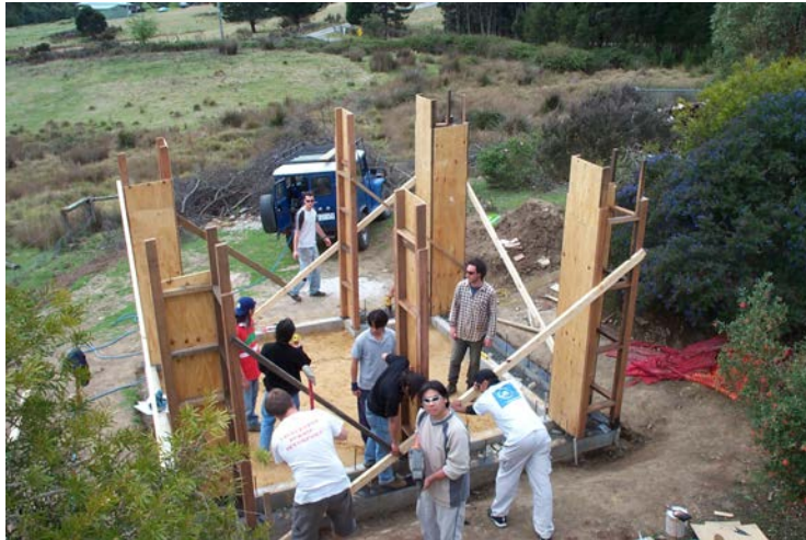
Image 11-8 Construction of frame by architecture students (Parnell, 2002)
