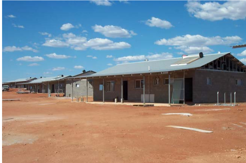
Image 10-6 New housing in Community 2, constructed under the National Aboriginal Health Strategy (NAHS) (Parnell, 2005)
