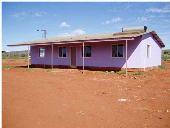
Image 10-3 House in case study community after renovation in 2005 (NT Government Department of Infrastructure Planning and Environment, 2005)
