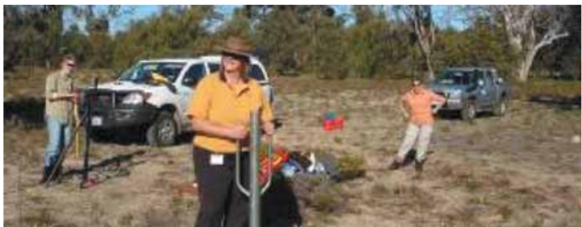
Building fences to protect restoration trials from kangaroos in Yalgorup National Park. From left: Amanda Hewison from Murdoch University, Lisa Wray from the City of Mandurah and Lyn O'Brien from the Friends of Island Point.
