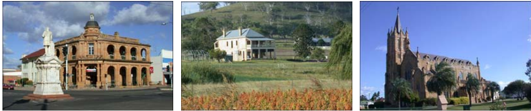
Figure 2.9 Cultural heritage is an important part of the Condamine Headwaters. Early buildings in the city centre and homesteads on farms are conserved and valued
