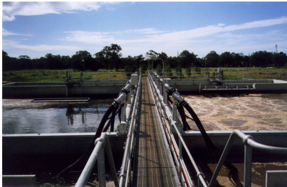
Figure 1.4: Two large-scale sequencing batch reactors treating domestic wastewater, operated in parallel (Busselton, Western Australia, ESI Ltd). The basin on the left was in the middle of the settle/decant phase, while the right basin was in the middle of the aeration phase. The decanting devices are visible at the far end of the basins.
