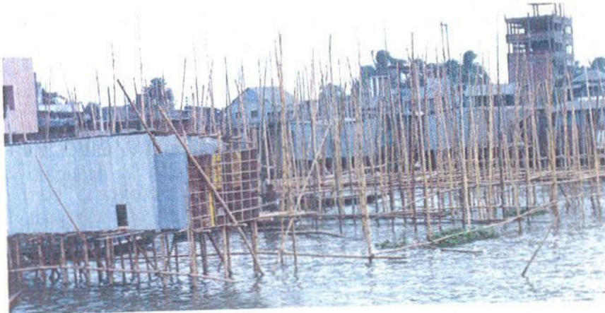
(b) Encroachment by traders/businessmen
