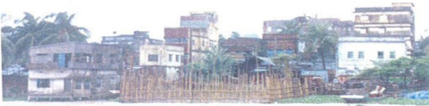
(a) Encroachment by resident houses
