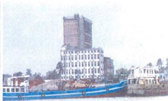
(b) Pollution by loading and unloading of building materials
