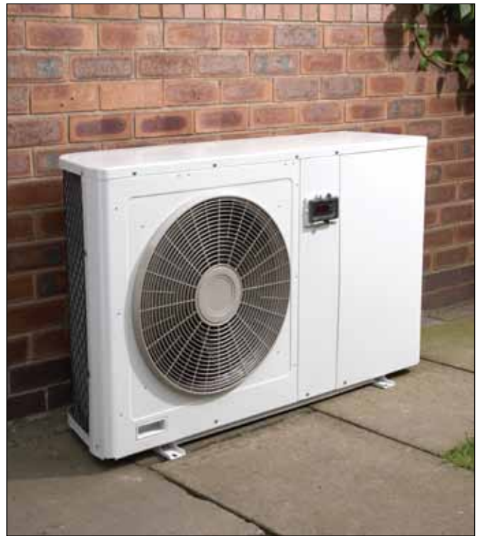
Sizing and positioning a heat pump are critical to running efficiency
