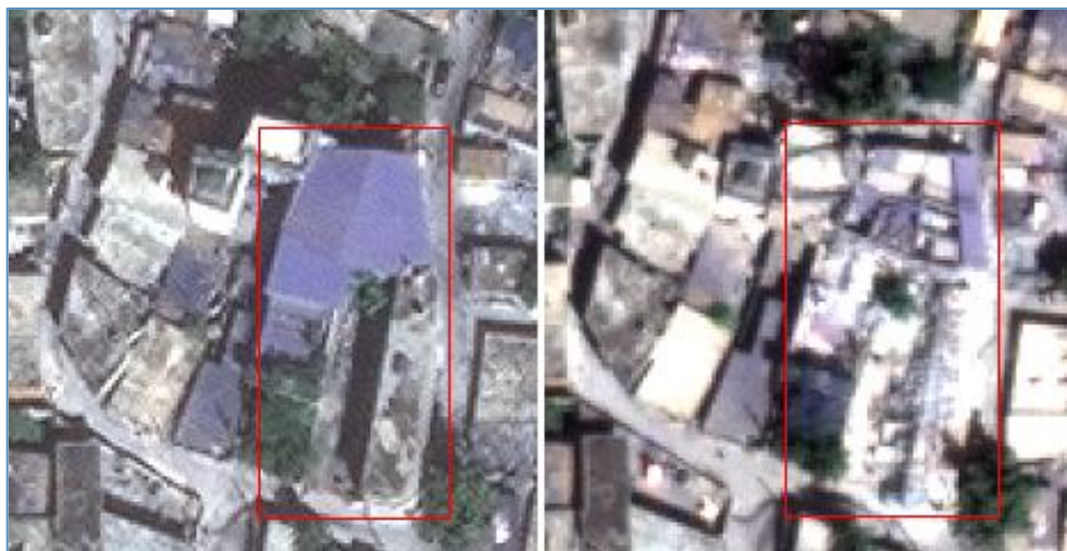
Figure 3.4: Pre- and post-disaster comparison of a collapsed building in Carrefour
