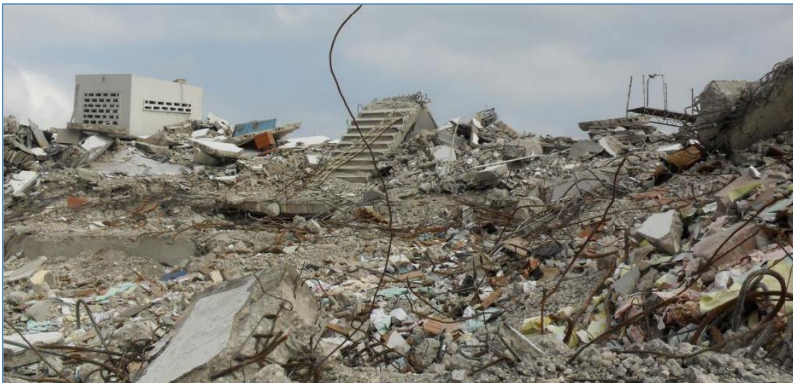
Figure 2.4: Complete destruction of a concrete building in Haiti
