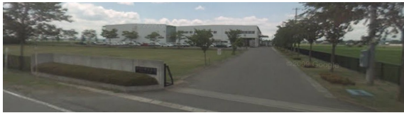
Figure 3. Image of the building reconstructed by means of SAR tomography (©Google). Its height can be estimated at 15 m - 20 m.
