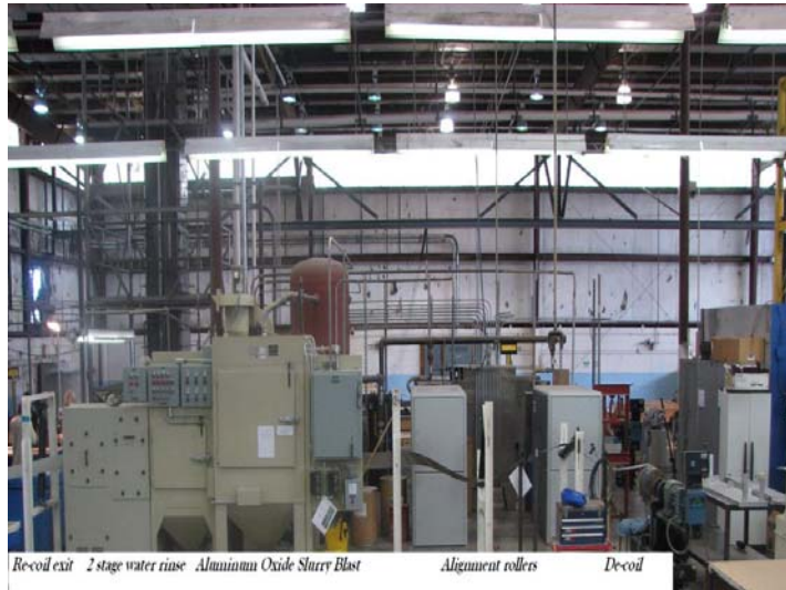
Fig. 3.4: MOD-1: slurry grit blast.
