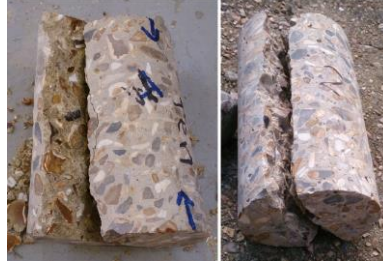
Figure 5, Core samples with satisfactory failure.
