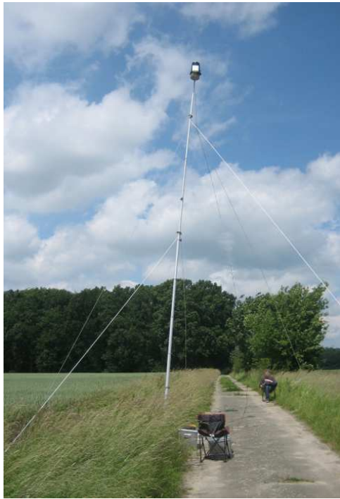
Figure 5. Pole mounted weather sensor system
