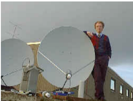
Figure 3: 1.2m satellite antenna after installation at a Partner Site.
