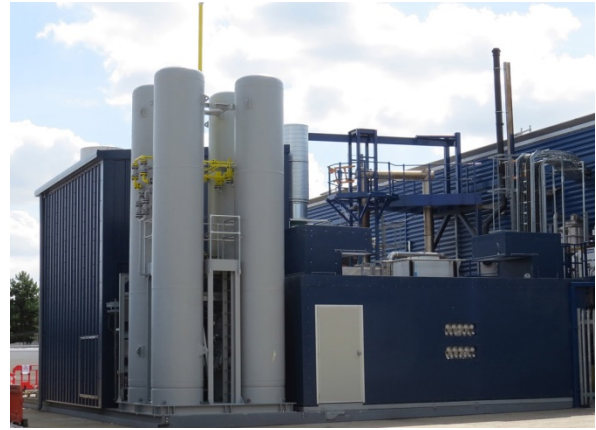
Figure 11: Direct photo of major components of the pilot plant: two-stage fluidised bed and plasma converter for syngas generation (left), syngas storage vessels and bio-SNG facility (right).
