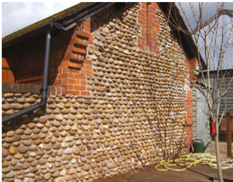
Figure 13.3b Pebble barn with brick quoins: The Warren, on the western side of the Pebblebed heathlands (Source: author)
