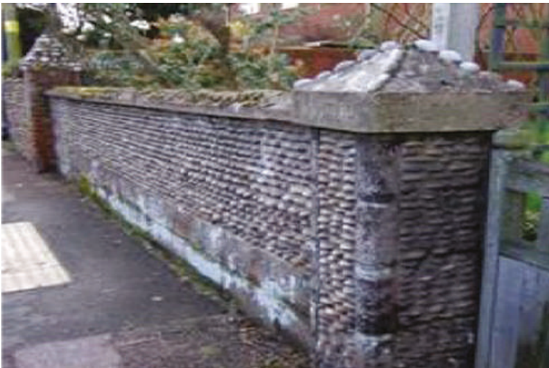
Figure 13.5d Woodbury: pebble wall with limestone topping (Source: author)
