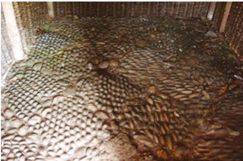
Figure 13.2b The pebble floor in the 'Bear Hut' in the grounds of Killerton House, Cullompton (Source: author)
