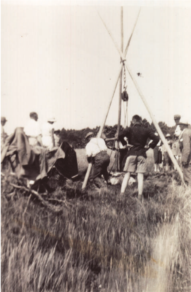
Figure 2.3b Lifting the stone (Source: Carter archive)
