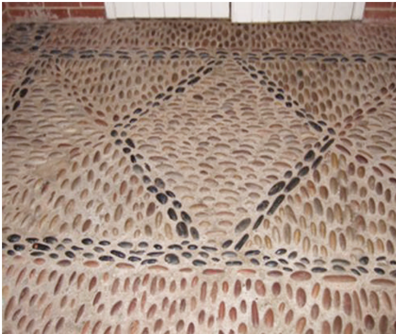
Figure 13.2c Aylesbeare village hall: entrance lobby with a pebble ‘mat’ in a diamond design (Source: author)
