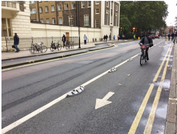
Figure 4: New cycle lanes in Bloomsbury, London, have been added following the removal of vehicle lanes (Matthew Carmona)
