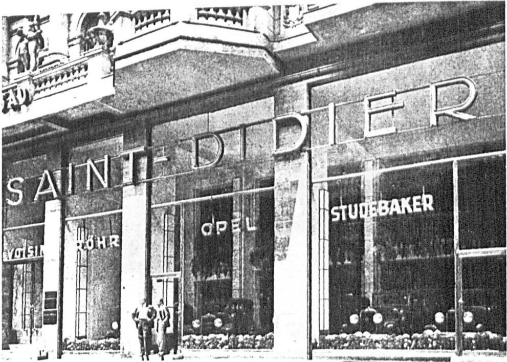
Fig. 58 Photograph from Das Neue Berlin of a car showroom on the Kurfürstendamm. Note the old elaborate ornamentation on the first floor above the modernized ground floor facade.
