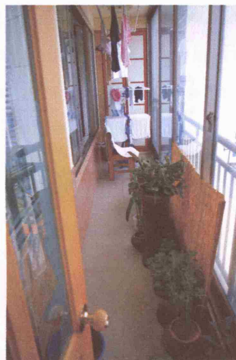
(b) Refurbished front balcony
